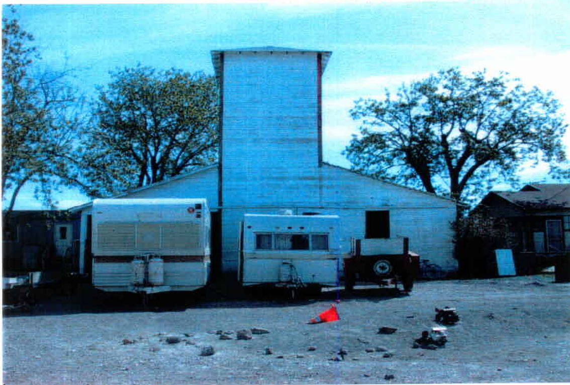
Photograph No. 5. View of old well/pump house used to provide drinking water to the residences living on the Mistler property. Tower of building previously housed a water storage tank.
