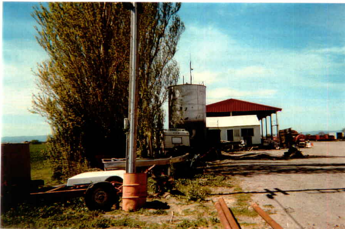
Photograph No. 10. View of 55-gallon drum (appeared to be full of spent motor oil) and diesel AST (approximately 10,000 gallon) seen in background and in center of Mistler property looking west. AST has a pump and dispenser attached to it. According to the property owner the AST is no longer being used.
